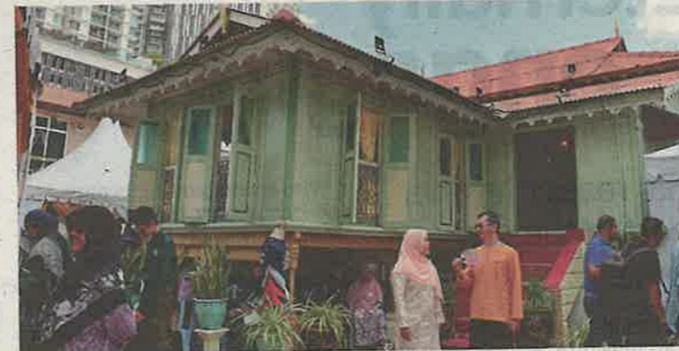
Villa Sentosa, the only surviving traditional Malay home in Melaka, is now a century old. — Bernama
