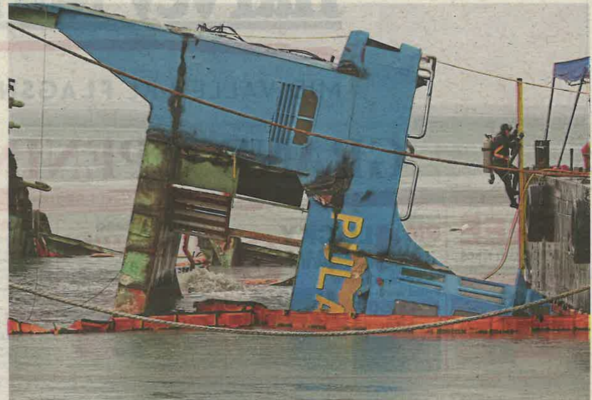
Arduous work: A diver preparing to go underwater to cut up 'Pulau Kapas' at the Butterworth wharf. — CHAN BOON KAI/The Star
